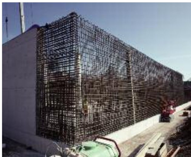
Water supply grid work at Kingston St Mary
