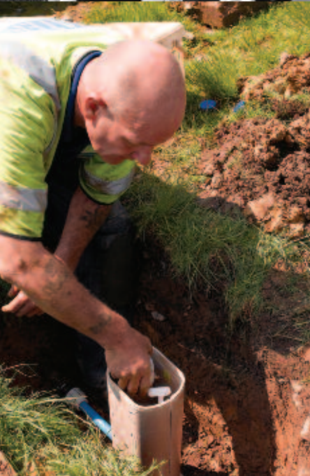
Meter replacement to a livestock trough in a field, left, and far right, and staff complete a waste transfer note, right.
