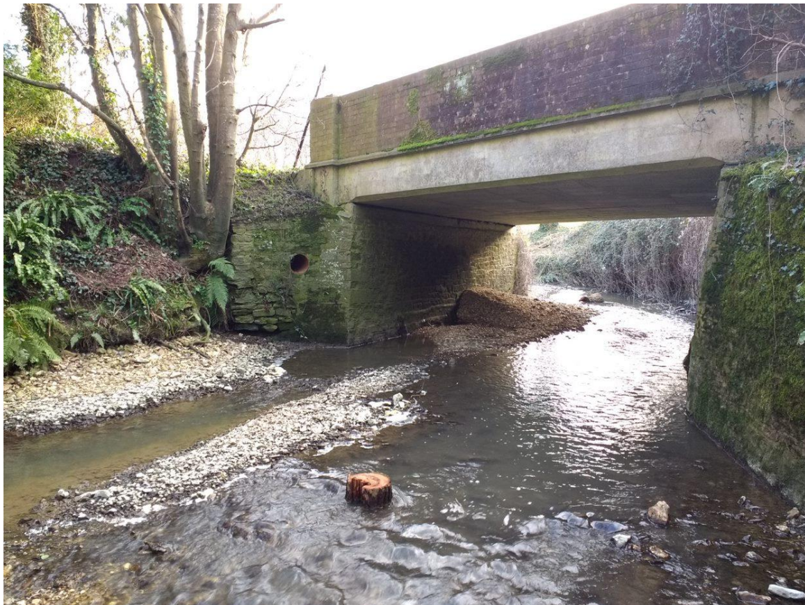
Figure 26 Downstream Yeovil reservoir, showing sediment introduced in AMP6 trial, 2019.
