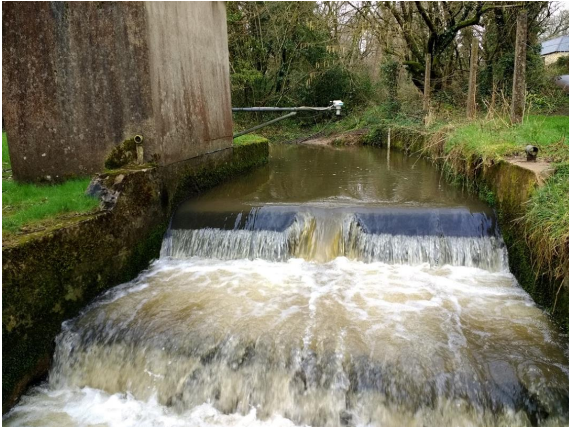
Figure 25 Knacker’s Hole gauging station, a barrier to fish passage.
