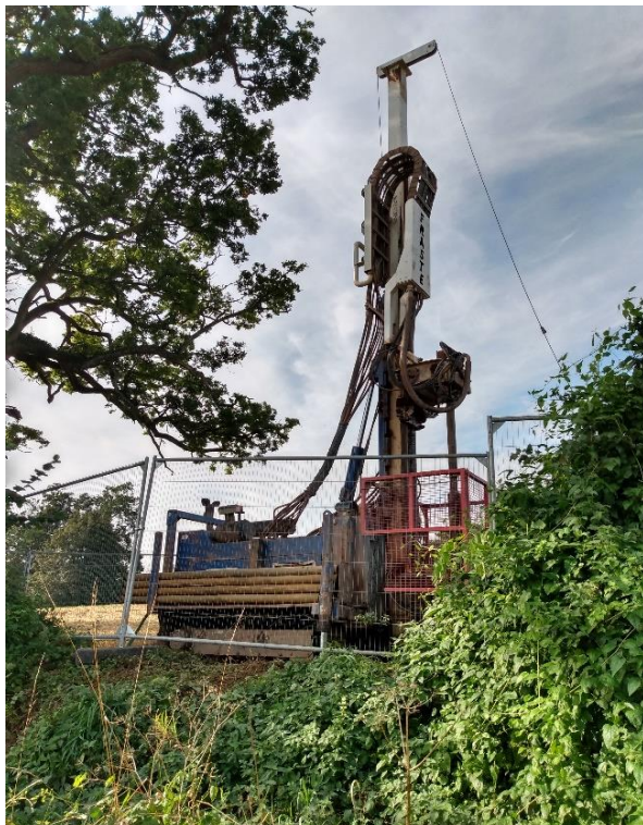
Figure 20 Geological explorations as part of our AMP7 Middle Bristol Avon groundwater investigation. Drilling rig (left) and retrieved geological core (right).
