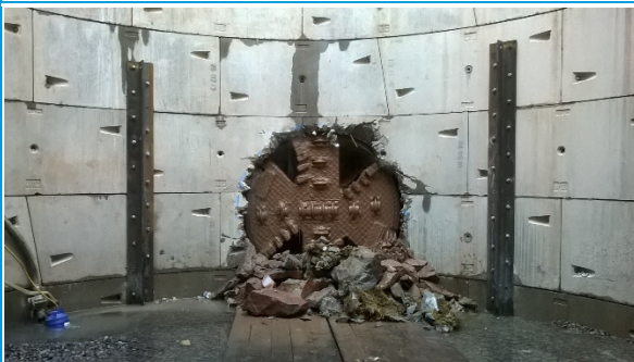
Tunnel machine breaking into shaft
