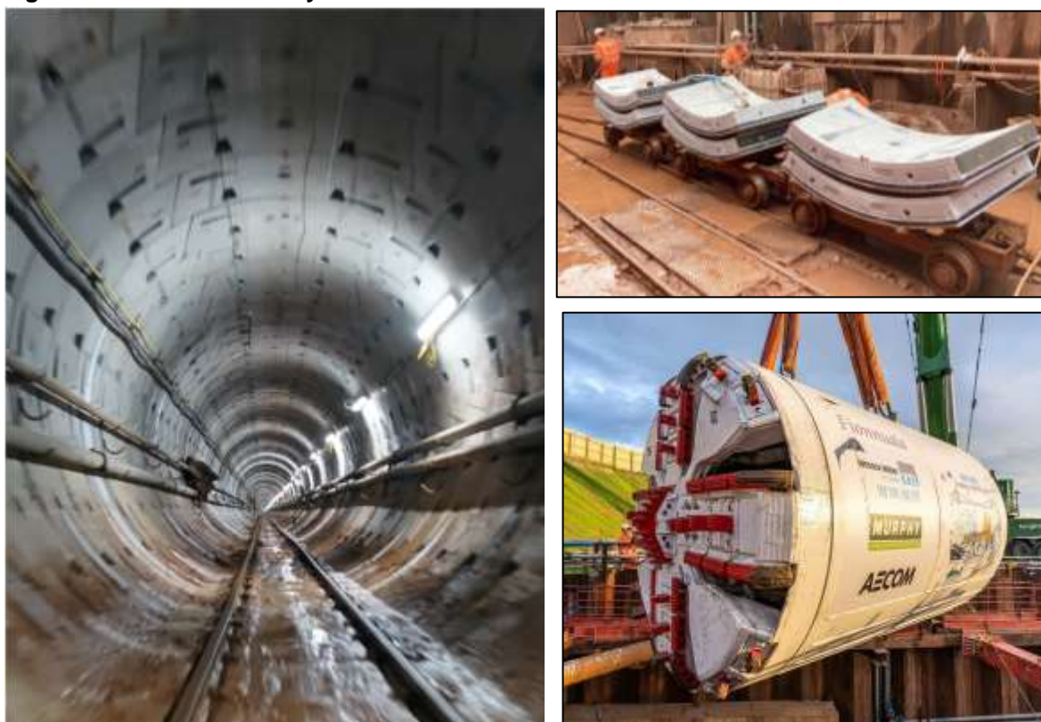
Figure 5: North Bristol – Trym sewer under construction
