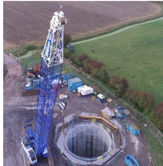
Picture 2: New storage shaft at new SPS
