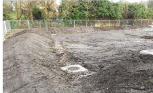
Enabling works (WW)
